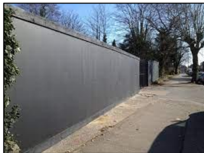
Plate 1: Example of Wooden Hoarding
